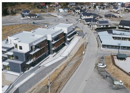
再建された研究実験棟と共同利用研究員宿泊棟 Reconstructed main building of International Coastal Research Center and the Guest House.
