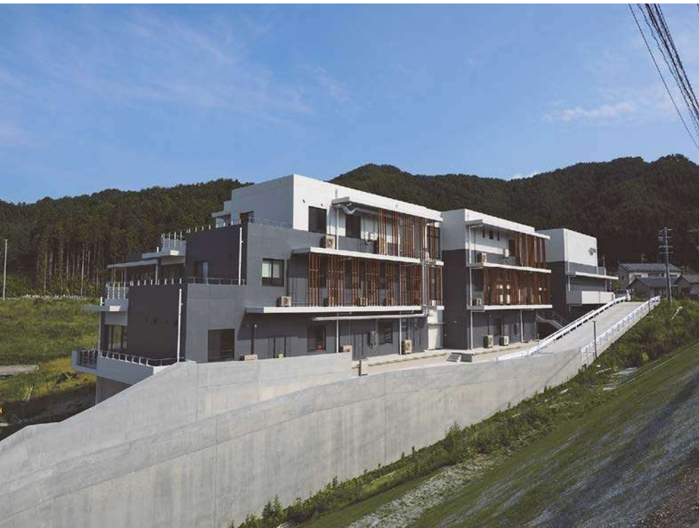
Photo 2. The new ICRC building and dormitory, completed in February 2018
